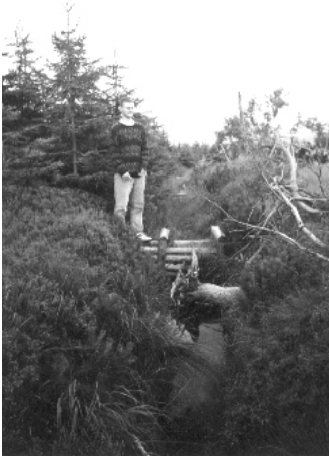
Fig. 4: To start spruce bog forest regeneration, palisade dams sealed up by peat were used to block draining ditches in the Giant Mountains.
